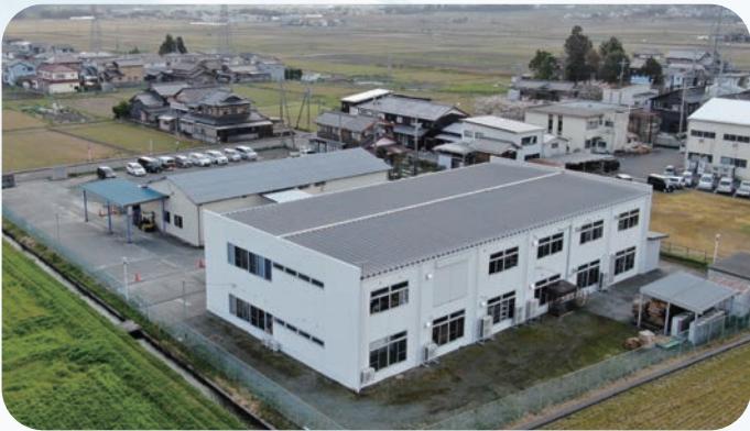
Shiga Factory (Shiga prefecture)
